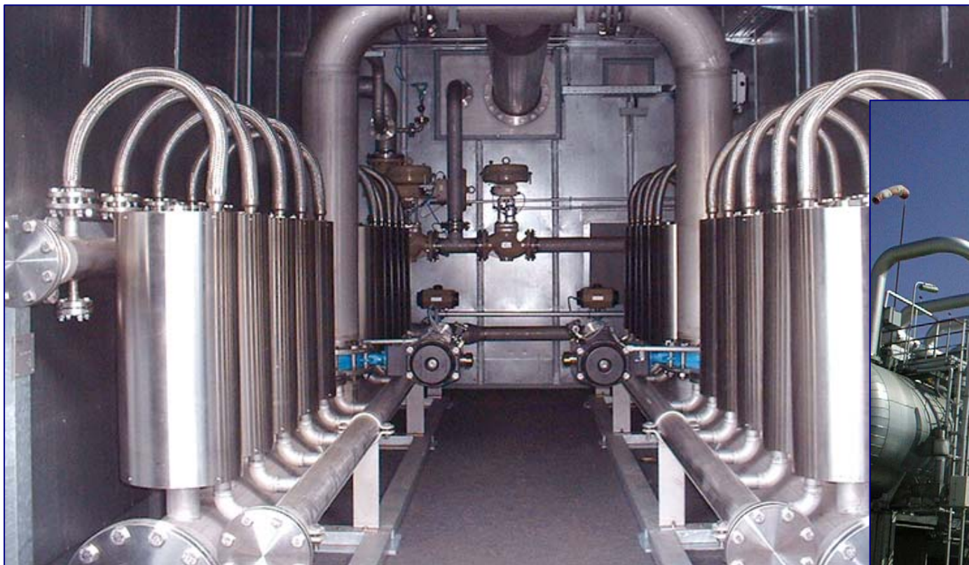
Inside view of a container-based membrane unit
